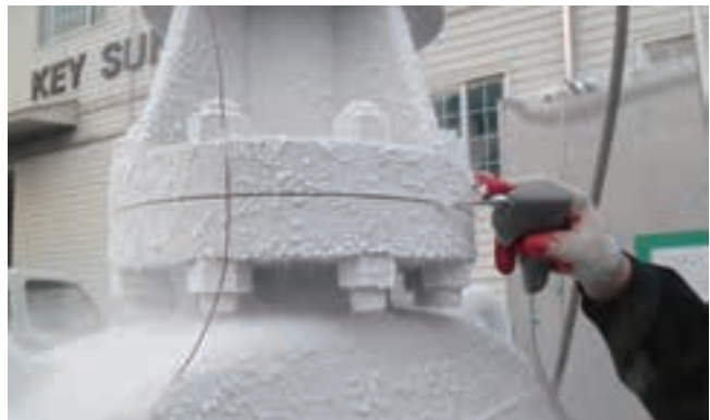
- Gasket leakage test
